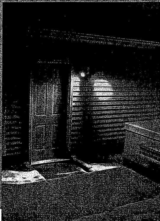
This residential security fixture, model SL-5597 by Heath Zenith, is one of the few to offer shielded bulbs. It also features motion-sensor activation and dual-brightness illumination.
