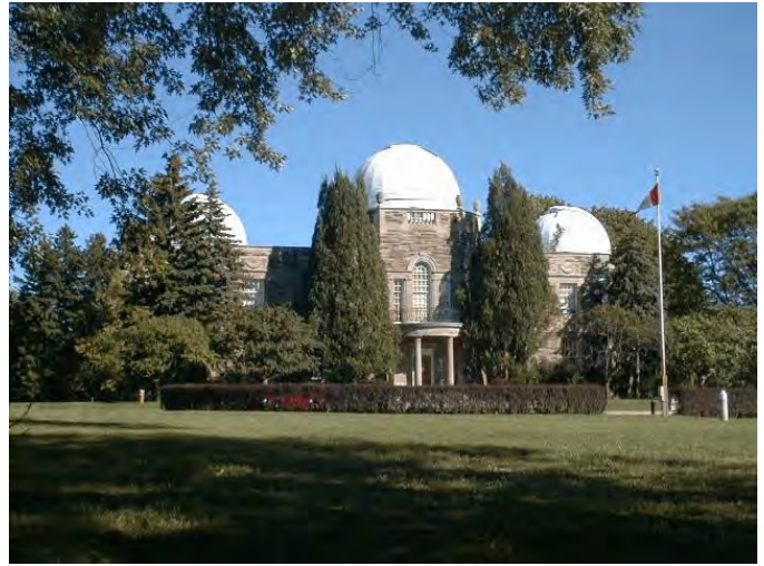
Figure 3 — The west administration building at the DDO.
