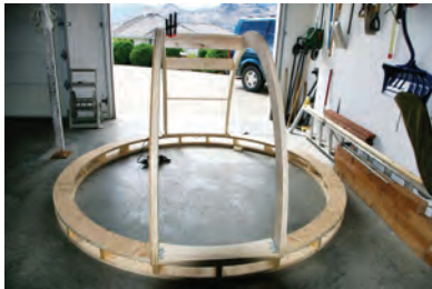
Figure 5 — Rings for base of Dome and centre supports.
