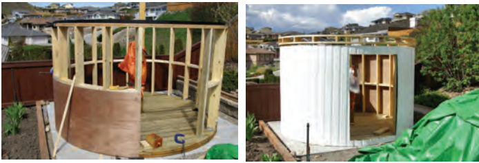
Figure 10 (left) — Applying 1/4-inch mahogany plywood Figure 11 (right) — Finished wall with vinyl siding and the dome base ring in place. Note the fence on the top of the wall, constructed at the insistence of my wife so that I would not fall again.
