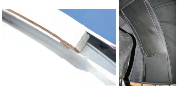
Figure 14 (left) — Rib of shutter door with aluminum strapping under lip of dome centre rib. Figure 15 (right) — Shutter with pulley system
