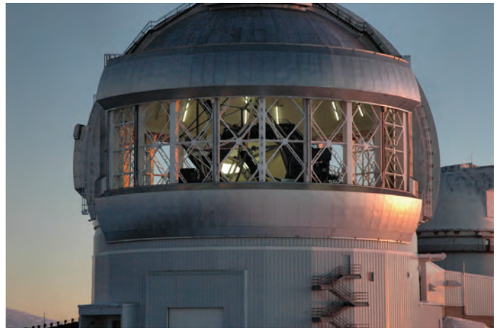
Figure 6 — Gemini opens to begin another night of discovery. The observatory opens along the side to allow a flow of cool air into the dome.
