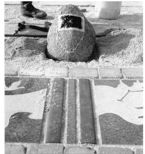
Figure 5 — Pair of rails marking local noon, separated by 15 cm to form the "noon gap" (photo Barrie Burnett)
