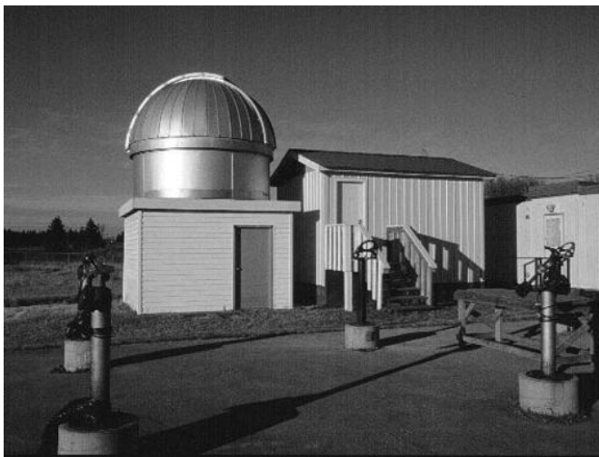
Winnipeg Centre's Glenlea Observatory
